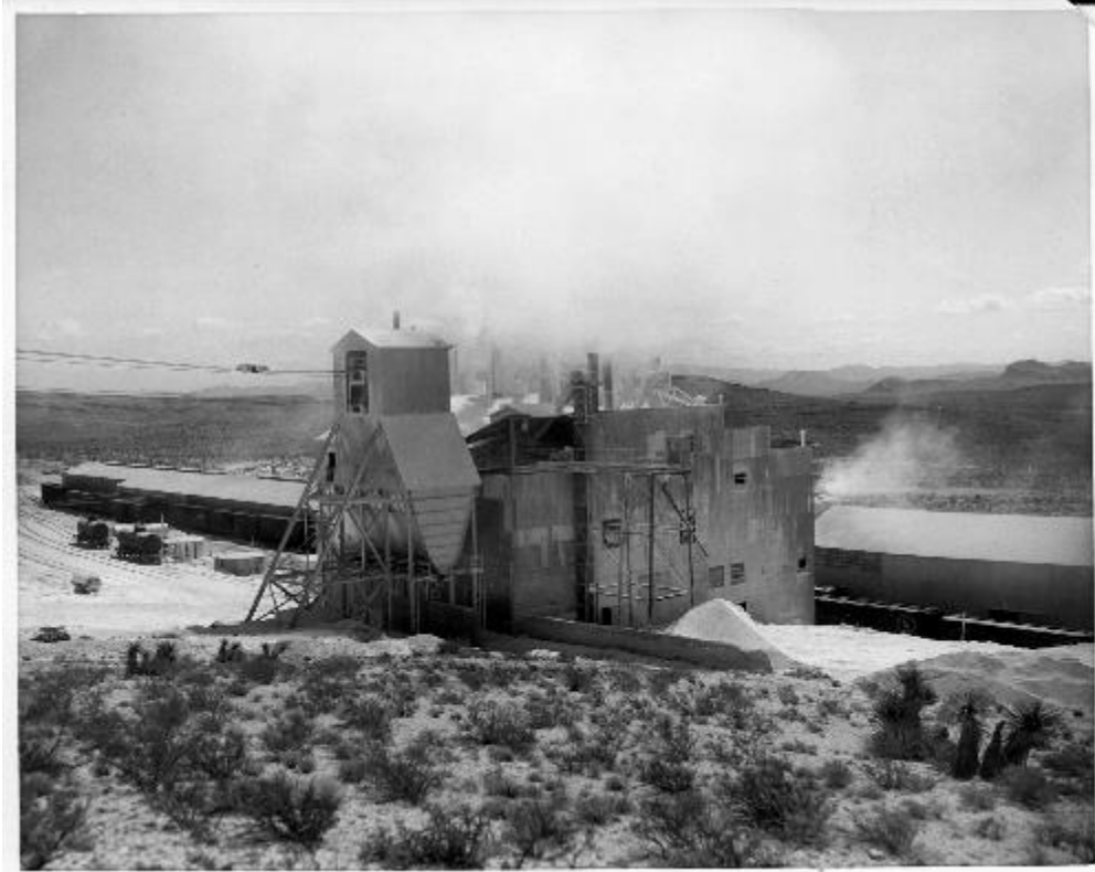
Blue Diamond Mill and Ore Loading Facility, from https://www.reviewjournal.com/uncategorized/southwest-of-las-vegas-village-of-blue-diamond-upholds-nevadas-legacy/ accessed Nov. 11, 2023
