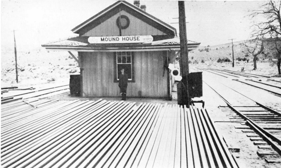
Caption: The Mound House train depot is seen here, in this view to the south. On the right is the standard-gauge Virginia and Truckee Railroad, and to left the narrow-gauge Carson & Colorado. From https://wnhpc.com/details/scttc0002 accessed Nov. 14, 2023.
