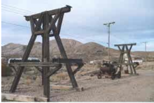
Figure 91. Darwin tram towers. By Gregg Wilkerson, 2003.
