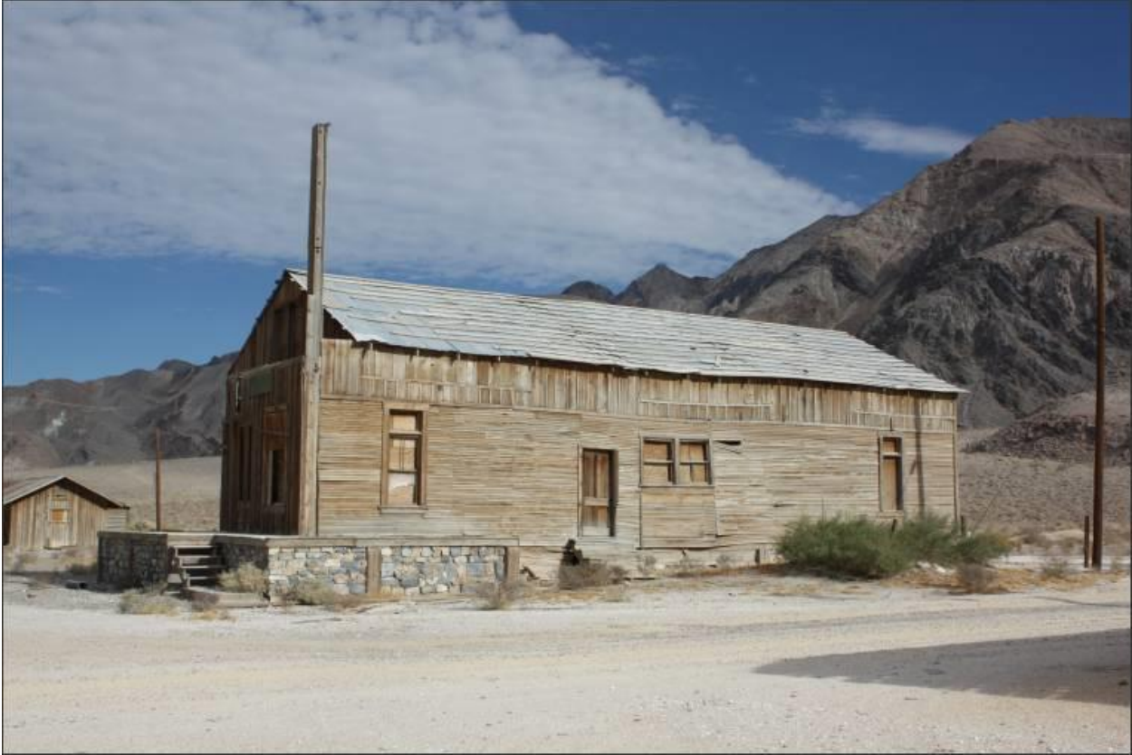
Figure 4. Abandoned building at Dolomite. From https://quarriesandbeyond.org/states/ca/quarry_photo/ca-inyo_dolomite_photos_2.html accessed March 3, 2024.
