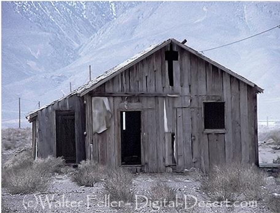
Figure 3. Although the above building at Dolomite appears to be authentic, it is not. It was originally built as a set for the movie, "Nevada Smith", starring Steve McQueen. Digital Desert; https://digital-desert.com/dolomite accessed March 3, 2024.
