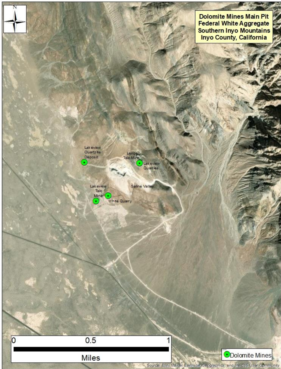
Figure 11. Aerial photograph of the main pit for the Dolomite Mines.
