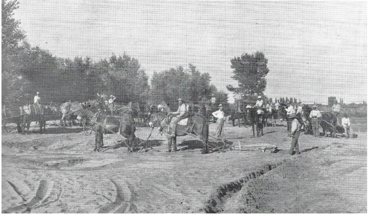
Caption: Owens Valley Railroad grade construction, 1911. From Frank Merrill photo, Arthur D. Haig Collection. From Myrick, 1962, p. 315.
