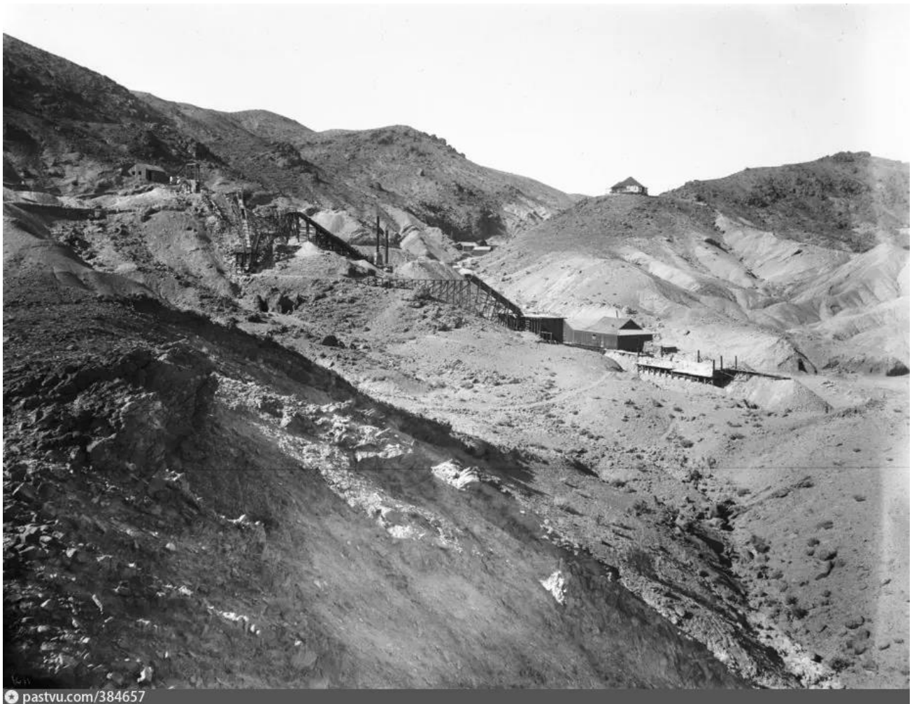
Caption: "Borax" Smith's mine, "Old Borate" ca.1890. Various buildings and equipment of the mining operation are situated in a rough line up the slope of the mountain. Smith's house is on top of the hill along the skyline. From Retro View of Mankind's Habitat; https://pastvu.com/p/384657 accessed Jan. 14, 2024,
