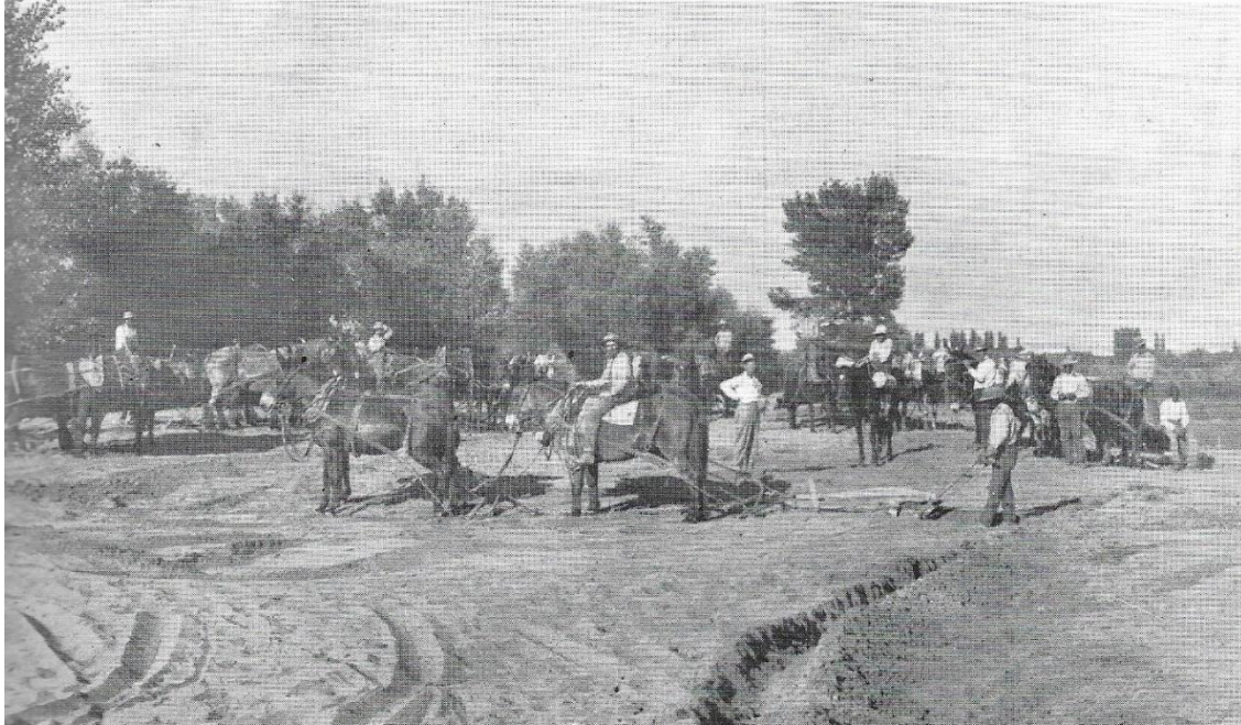
Caption: Owens Valley Railroad grade construction, 1911. From Frank Merrill photo, Arthur D. Haig Collection. From Myrick, 1962, p. 315.
