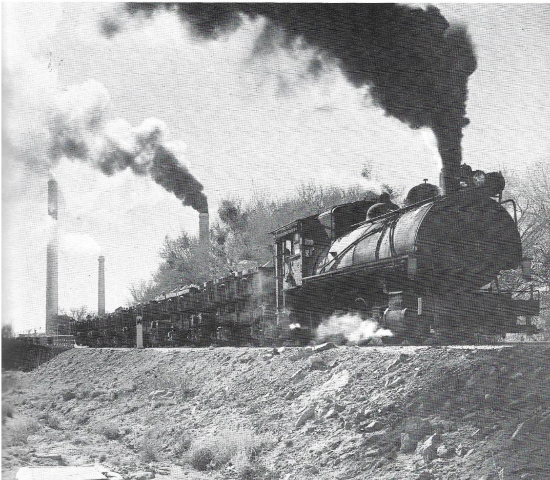
Caption: Mojave and Northern backing into Leon Plant. From Myrick (1963:865); Southwestern Portland Cement Company Collection.
