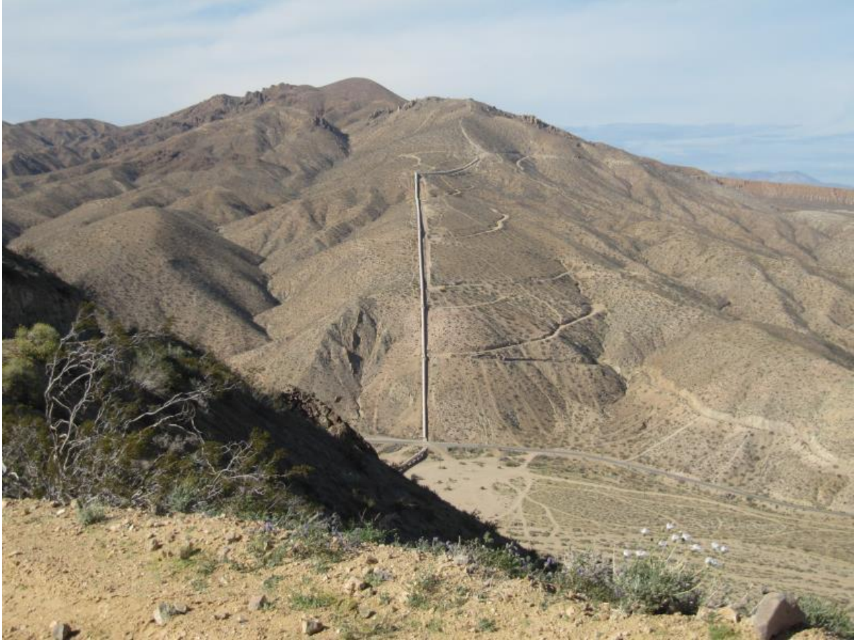
Caption: Los Angeles Aqueduct at Red Rock Canyon. From VenturaCountyTrails.org; https://venturacountytrails.org/RecentPhotos/2015-03-25RedRockCynSP/ Page.html accessed Feb. 11, 202.
