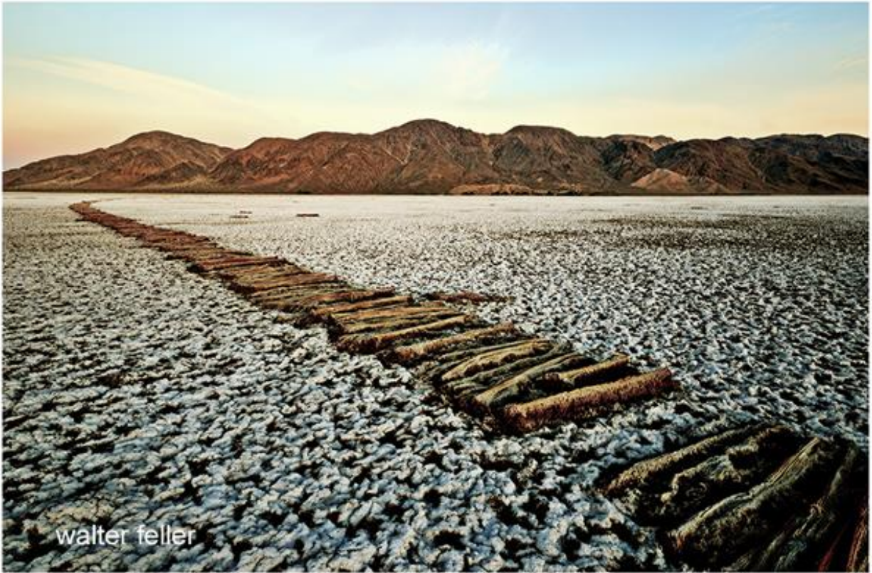
Caption: Soda Lake Railroad ties. By Walter Feller. From https://mojavedesert.net/railroads/railroads-061.html accessed Nov. 15, 2023.
