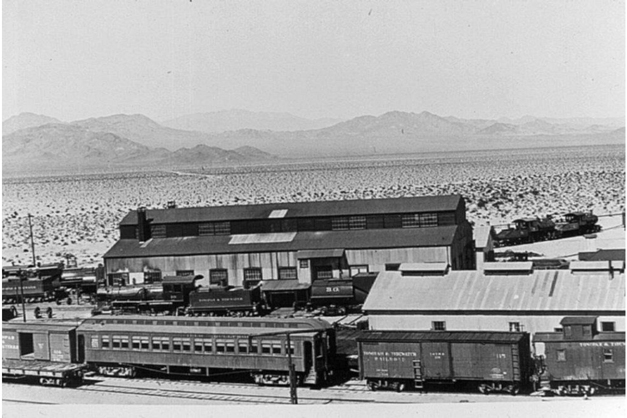
Caption: Tonopah and Tidewater station in Ludlow 3; https://pics66.com/pictures/8%20California/820%20Ludlow/Tonopah%20and%20Tidewater%20railway/index.html#img=Tonopah%20and%20Tidewater%20station%20in%20Ludlow%203.jpg accessed Nov. 11, 2023.
