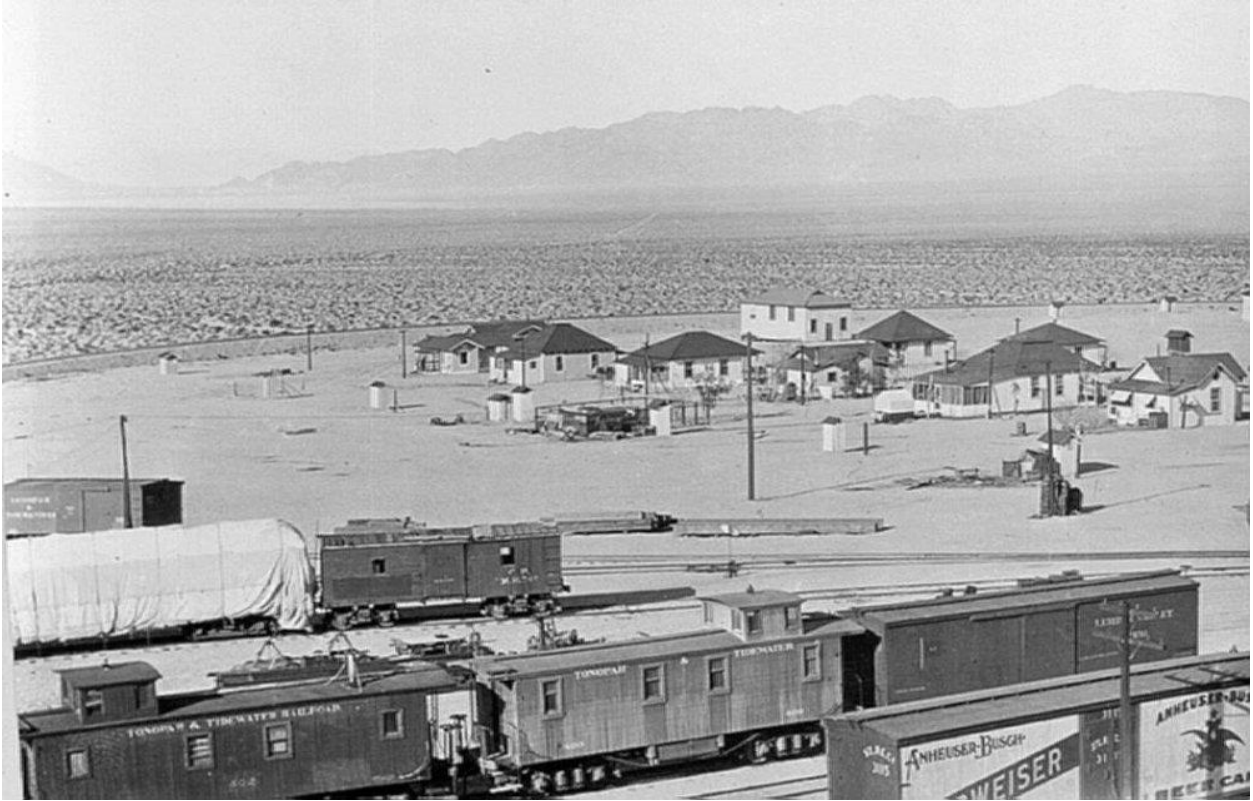
Caption: Tonopah and Tidewater station in Ludlow 4; https://pics66.com/pictures/8%20California/820%20Ludlow/Tonopah%20and%20Tidewater%20railway/index.html#img=Tonopah%20and%20Tidewater%20station%20in%20Ludlow%204.jpg accessed Nov. 11, 2023.
