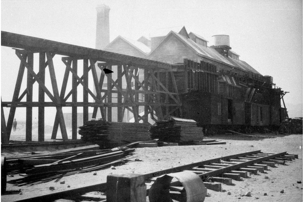
Caption: Pacific Coast Borax plant, Death Valley Junction. Photo by C. Marion circa 1900. From California State Mining Bureau Bulletin 11 Photo No. DM B7625a and From the Larry Vredenburg Collection No. 58e-02.
