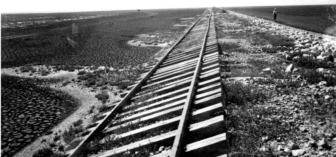
Caption: Abandoned track of Tonopah & Tidewater Railway across Silver Lake playa, looking south from near Silver Lake Station. Track was lifted from grade by flood waters in January, 1916. T. 15 N., R. 8 E. San
