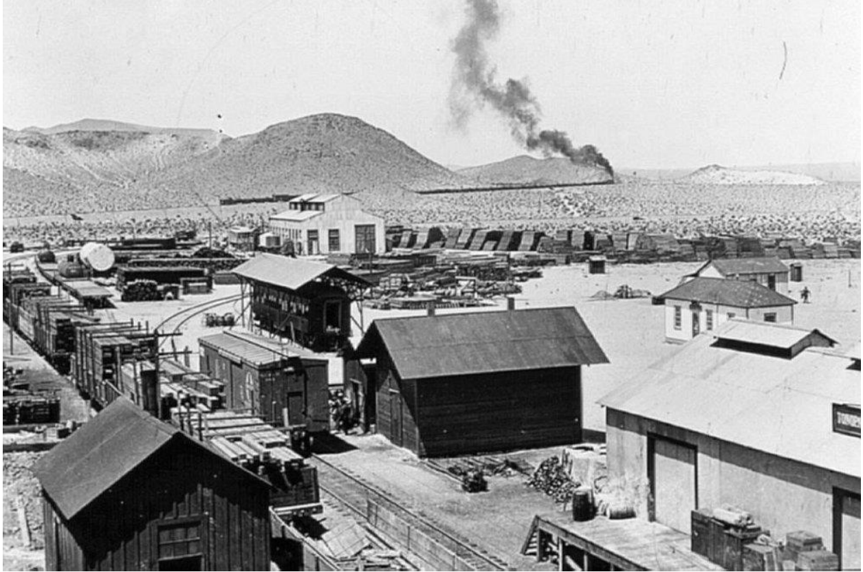
Caption: Tonopah and Tidewater station in Ludlow 5; https://pics66.com/pictures/8%20California/820%20Ludlow/Tonopah%20and%20Tidewater%20railway/index.html#img=Tonopah%20and%20Tidewater%20station%20in%20Ludlow%205.jpg accessed Nov. 11, 2023.
