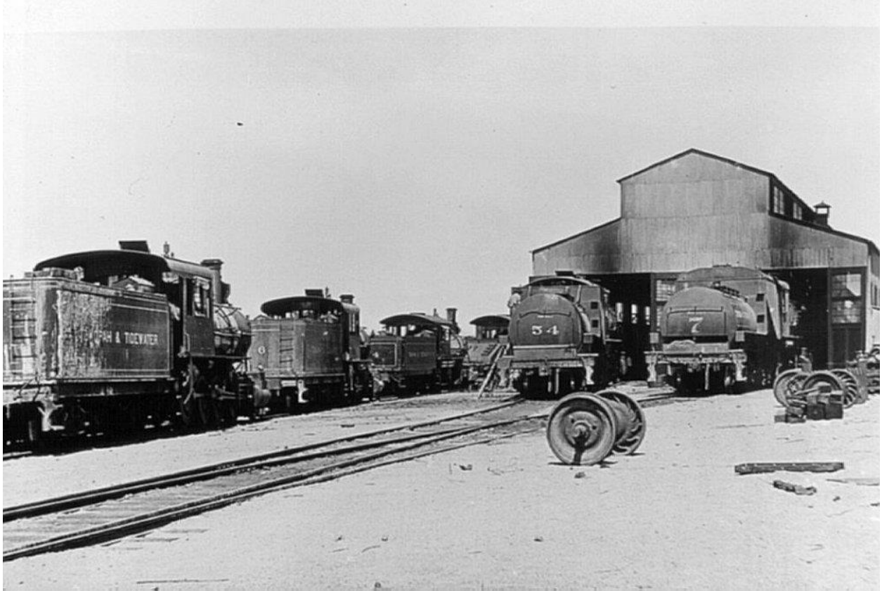
Caption: Tonopah and Tidewater station in Ludlow 8; https://pics66.com/pictures/8%20California/820%20Ludlow/Tonopah%20and%20Tidewater%20railway/index.html#img=Tonopah%20and%20Tidewater%20station%20in%20Ludlow%208.jpg accessed Nov. 11, 2023.
