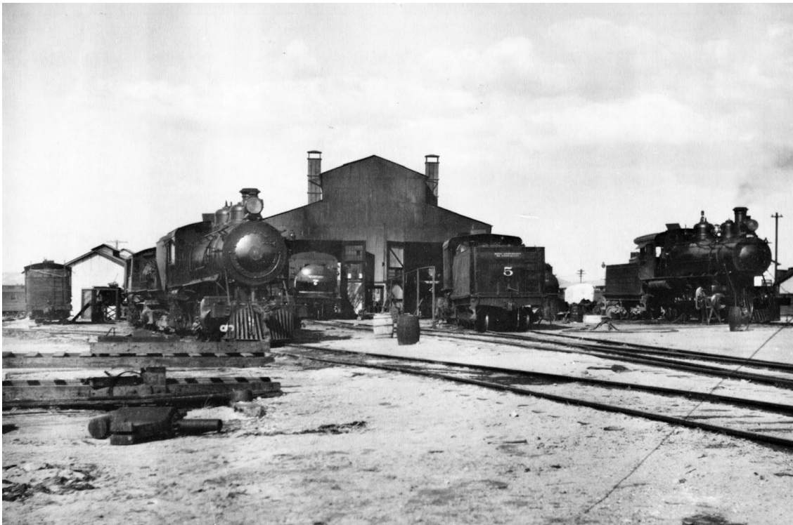
Caption: Tonopah & Tidewater engine house at Ludlow, California. T & T, and Bullfrog & Goldfield engines baking in the hot California sun. August 1909. Frank Green photo. D. L. Garcia Collection From 1981, California Southern Railroad Calendar.
