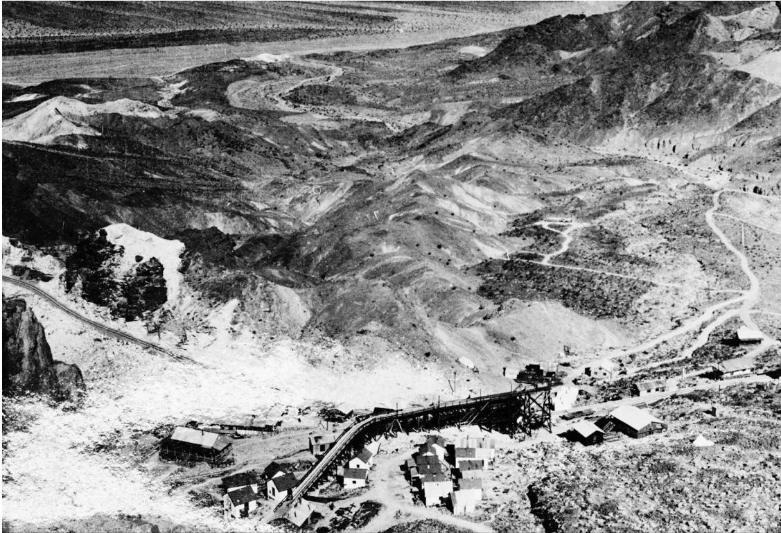
Figure 18. Ore bins at the town of Ryan. View is to the northwest down Furnace Creek. From the Larry Vredenburg collection.
