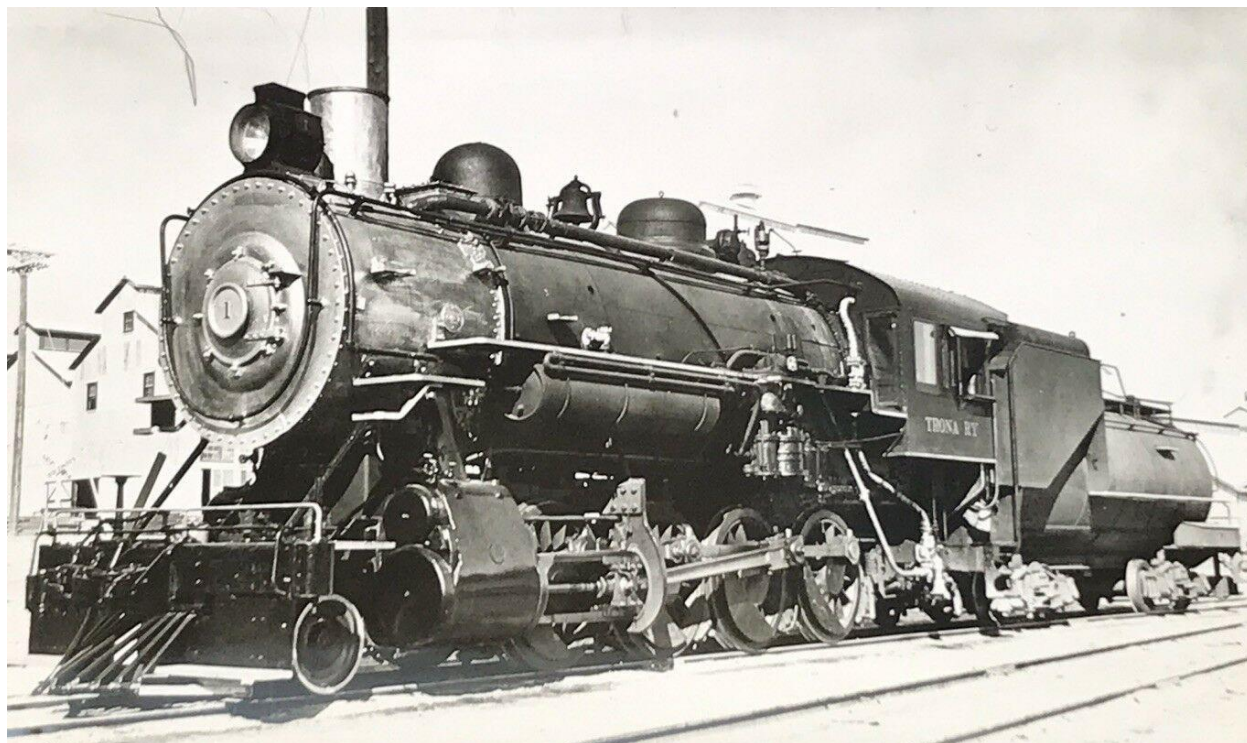
Caption: Trona Railroad Engine No. 1. at borate processing facility. From the Larry Vredenburg Collection.
